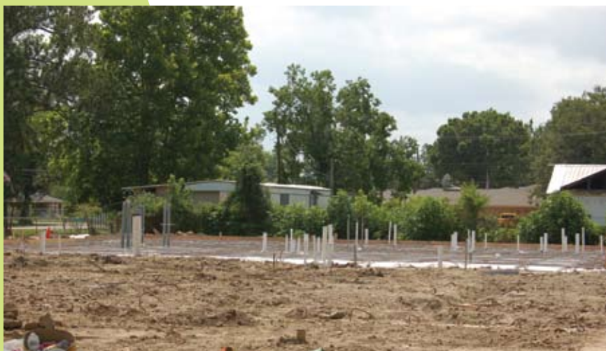
The foundation is complete on the new fire station.
