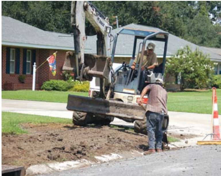
Shown are scenes from work to replace curbing on streets. A total of 20,000 linear feet of curbing will be replaced as part of the city's road improvement project.
