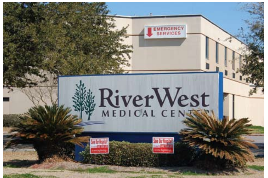
River West Medical Center, shown above, is currently closed, but parish officials are working to determine repair costs and get federal funding to repair and re-open the hospital.
