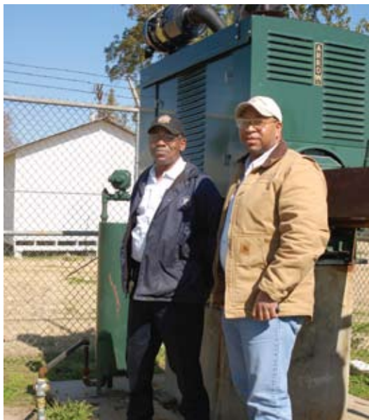
Town Maintenance Supervisor Lee Butler and Mayor John Overton are shown in front of the new engine that powers water well #2.
